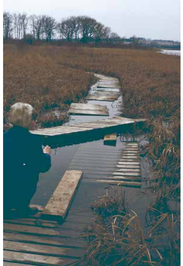
The wooden boardwalk required much maintenance, especially in flood years.
