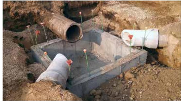
*This under-street catch basin, shown under construction, will capture debris from storm sewers and keep it out of the Yahara River and the lakes downstream. Photo by Jan Axelson.*
